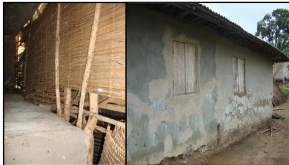
Inadequate Staff housing for health workers. Substandard construction with unfinished walls.
